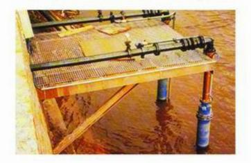
Since the Bottom Intake Pumps are suspended from the riser pipe without any other support they can easily be installed or removed.
